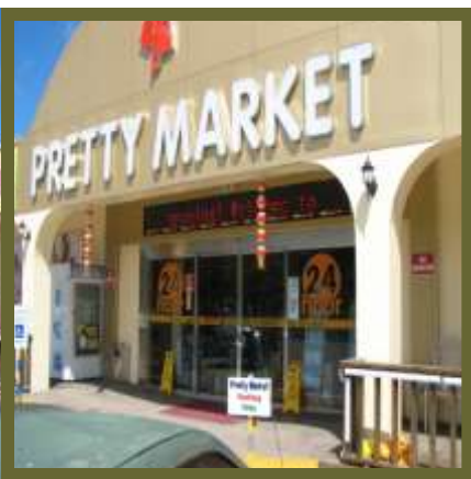
Above: New improved awning on building's exterior Right: Improved daycare facility with fenced playground, landscaping
